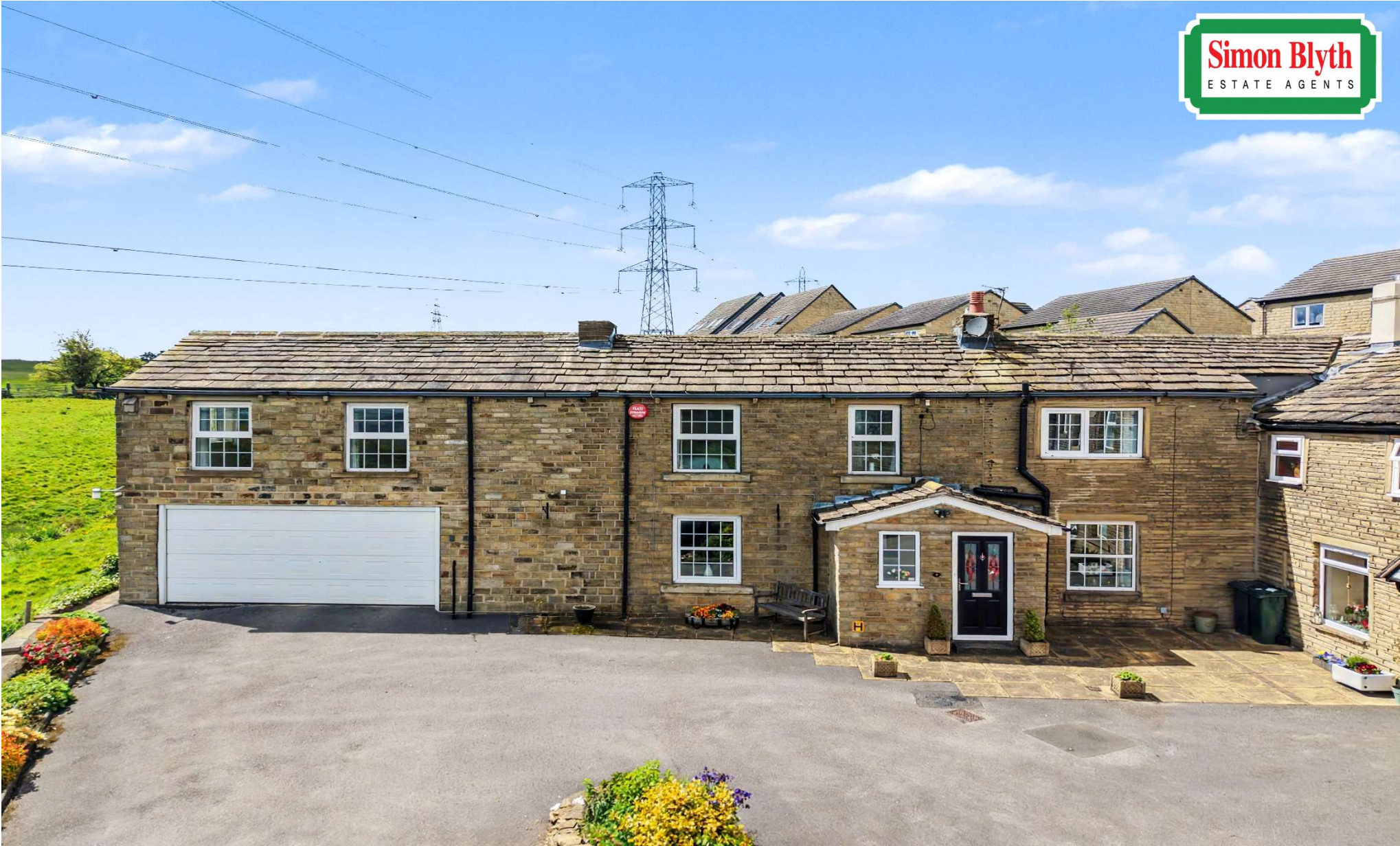
9 Warren House Lane, Lindley Moor, Huddersfield, HD3 3RS
