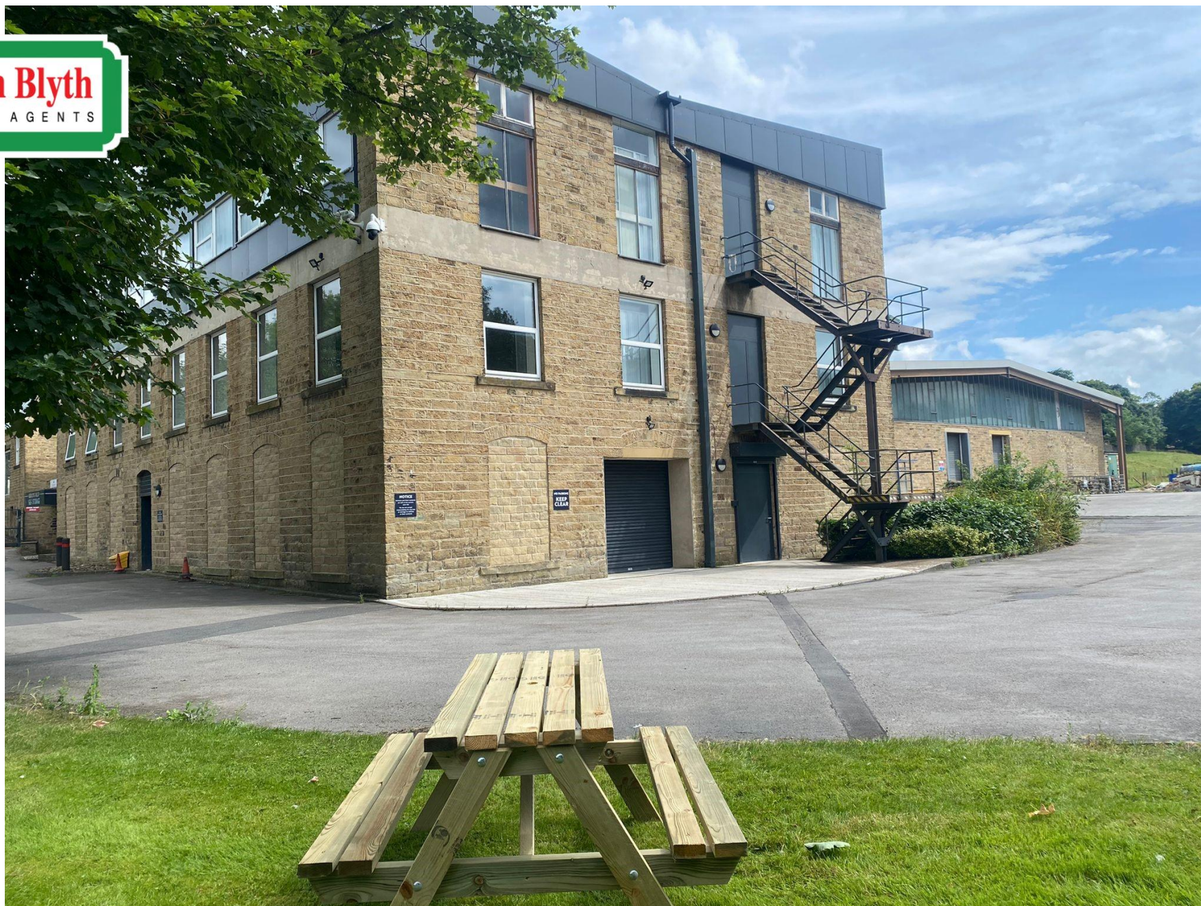
DOGLEY MILLS, PENISTONE ROAD, HUDDERSFIELD, HD8 0LE
