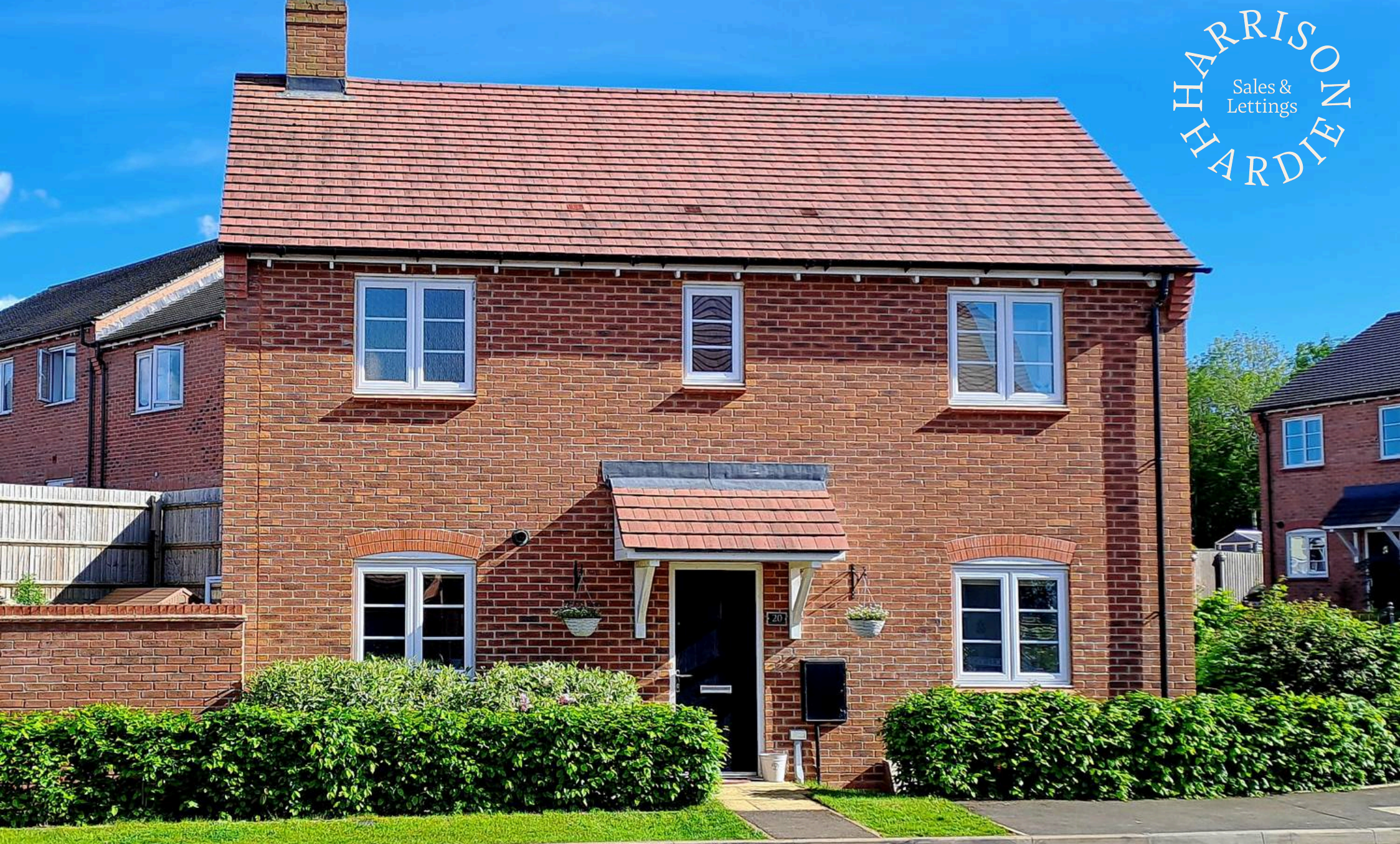
Norgren Crescent, Shipston-On-Stour
