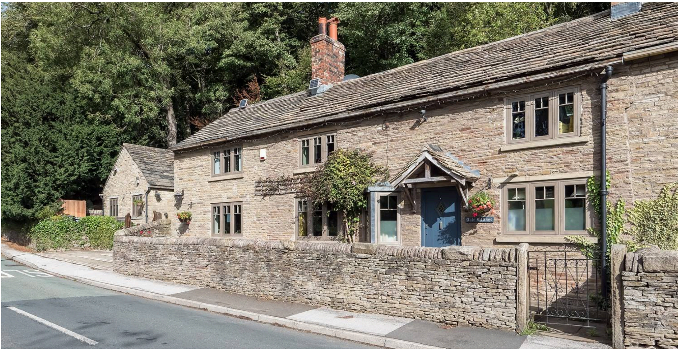
Vale Cottage Shrigley Road, Pott Shrigley
