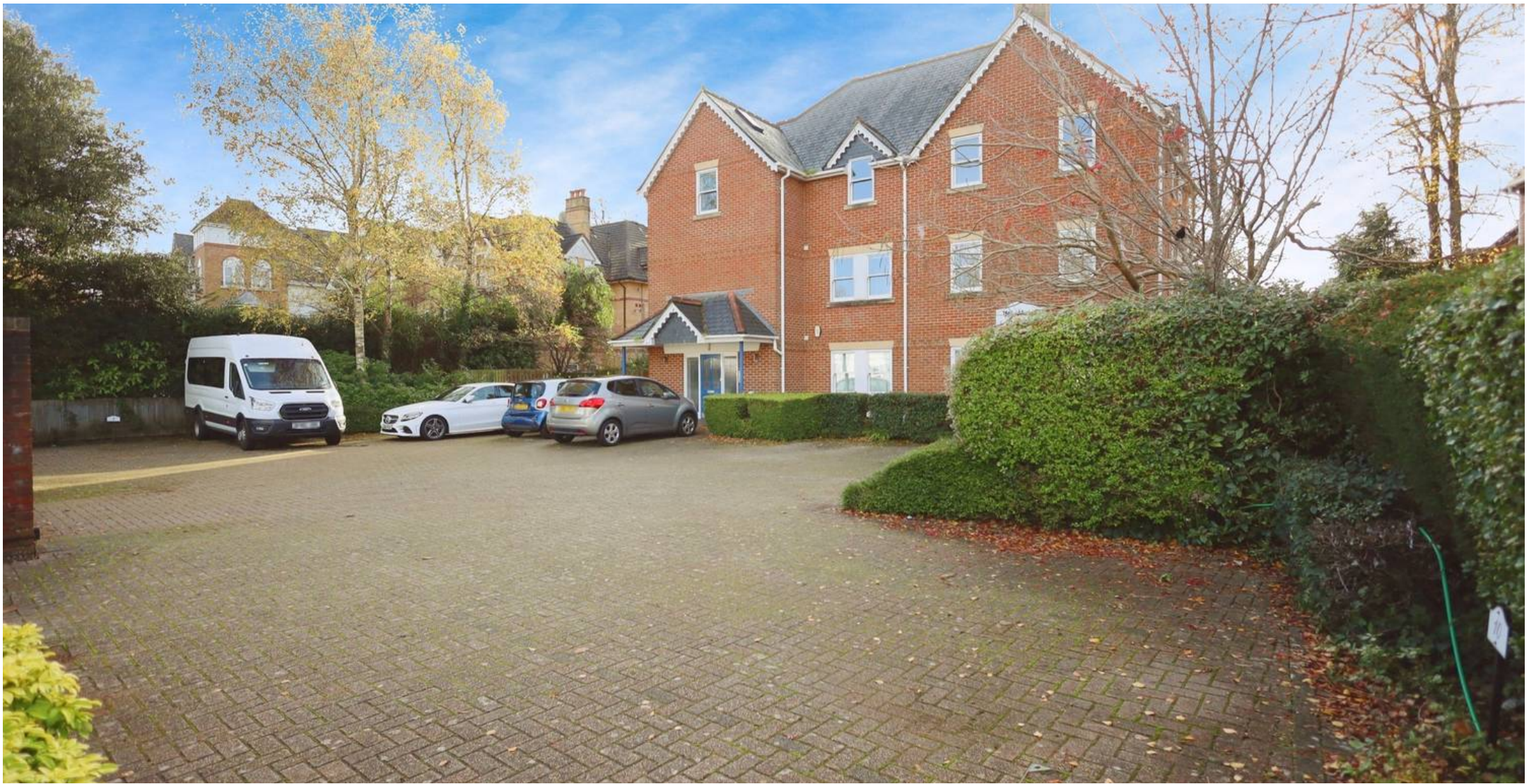
Flat 4, Westbury Grange, 62 Lansdowne Road Bournemouth
