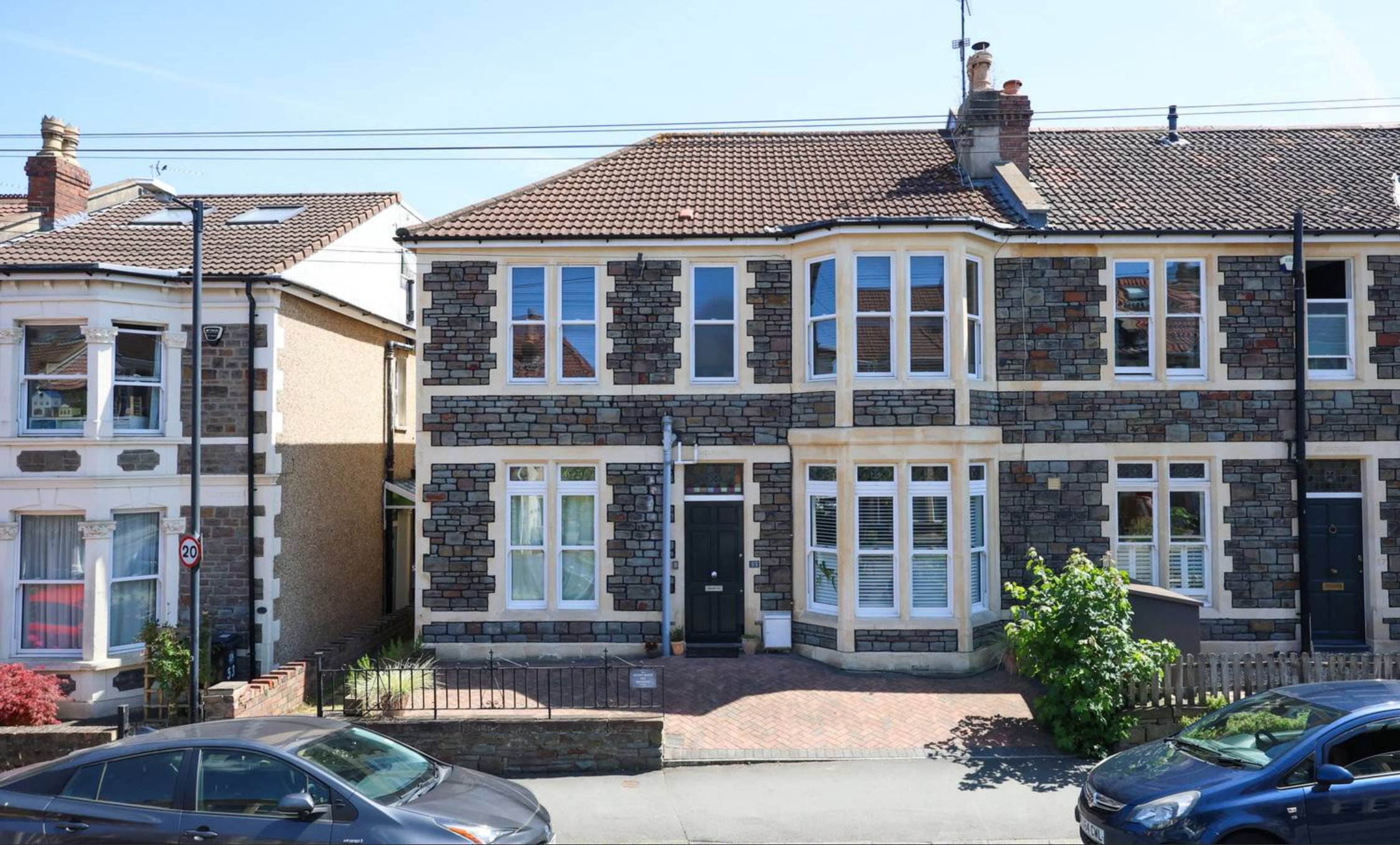
First Floor Flat, 55 Kennington Avenue, Bishopston £399,950
