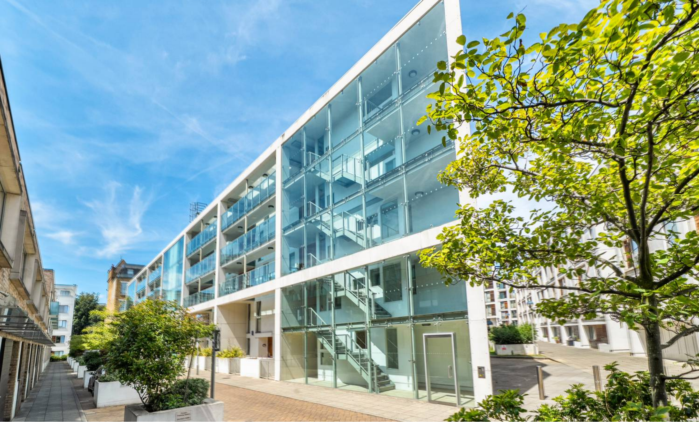
Flat 305, Causton House, 13 Printers Road £380,000
