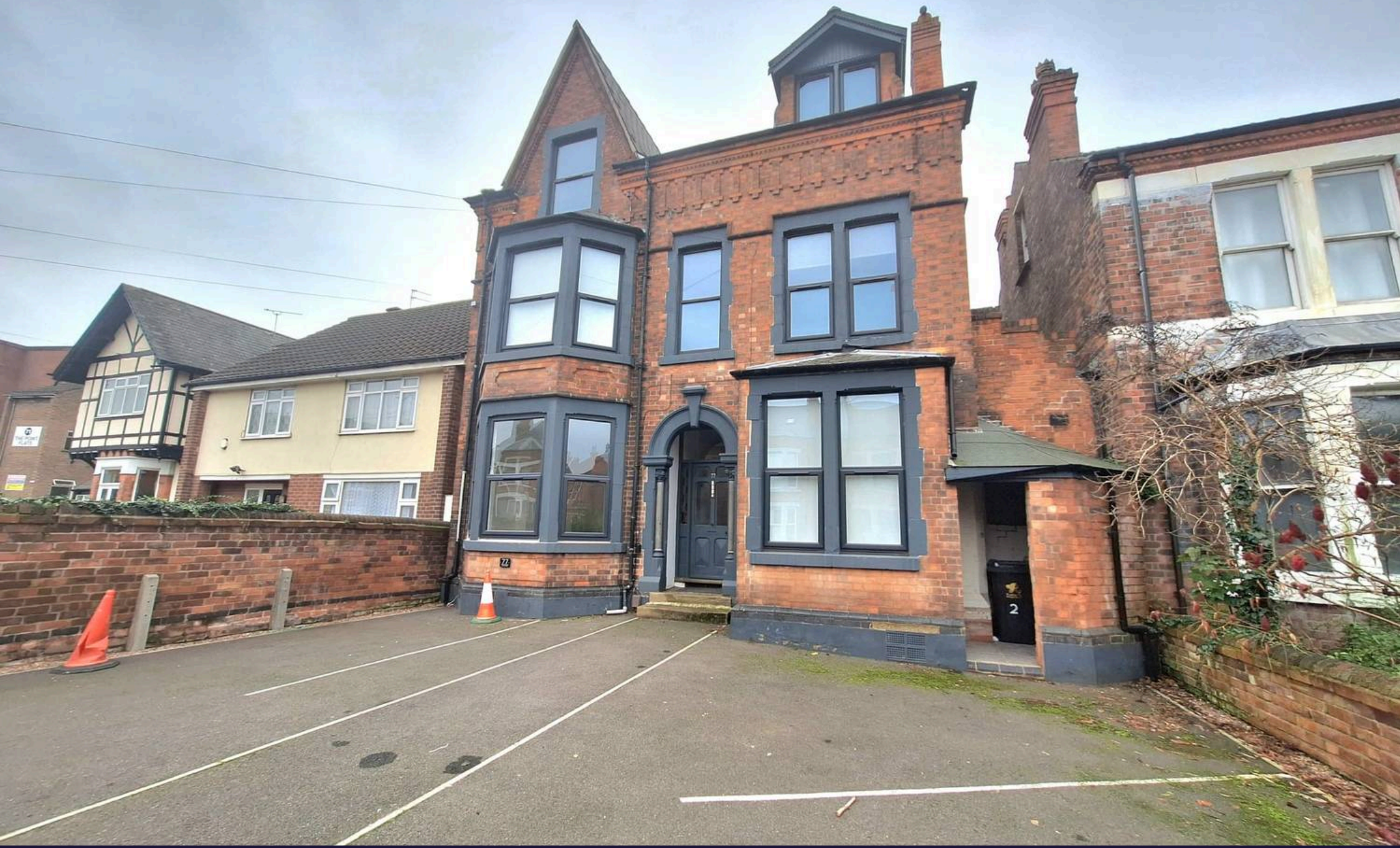
Flat 1, Loughborough Road, West Bridgford £895 PCM
