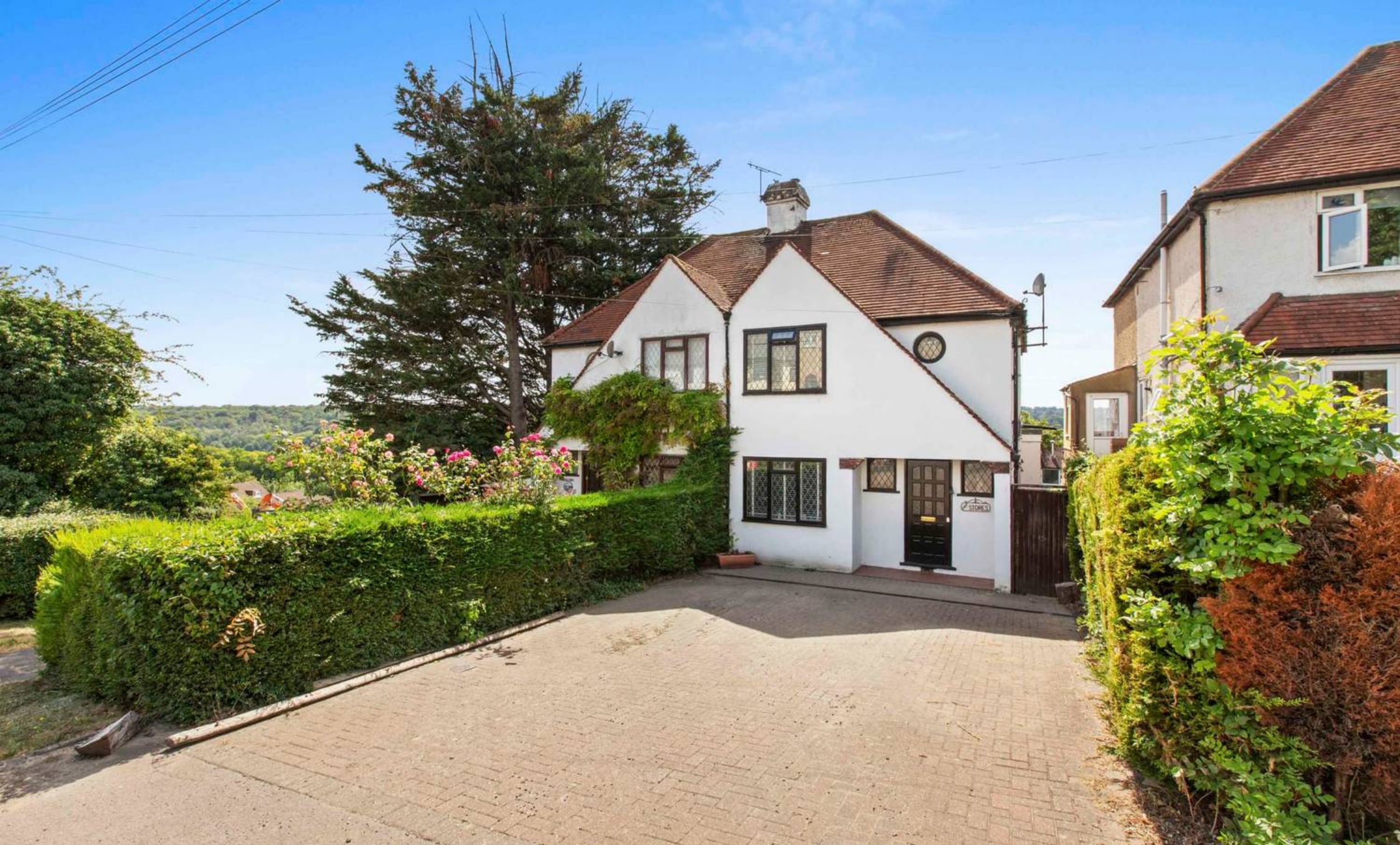
The Stores Hammersley Lane, High Wycombe - HP13 7BX £465,000
